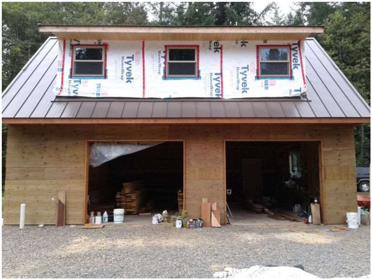
Figure 4: Partially Built Building That Started as a Carriage House and Would Become an Accessory Building
